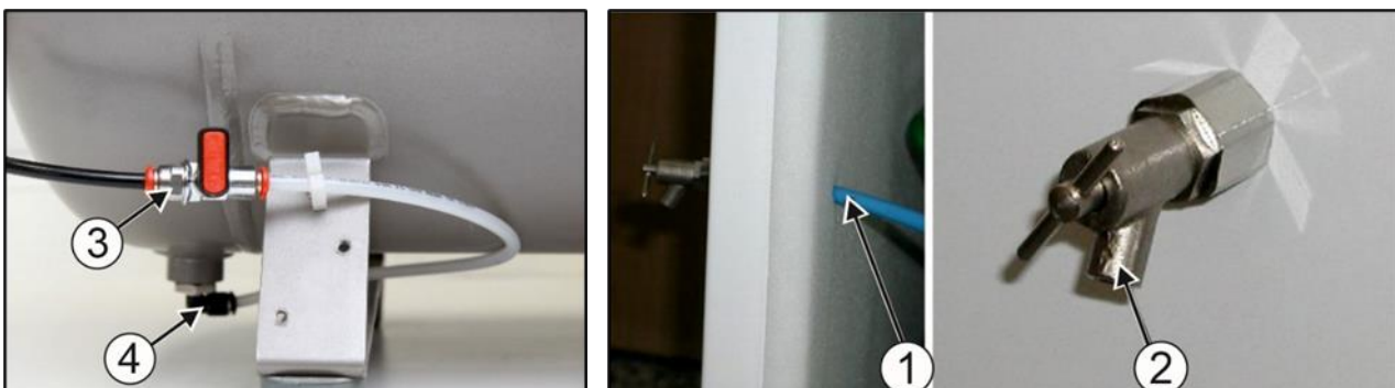
Fig. 7: Installation of condensate drain valve on cabinet
