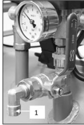
Fig. 8: Connecting to the compressed air outlet
