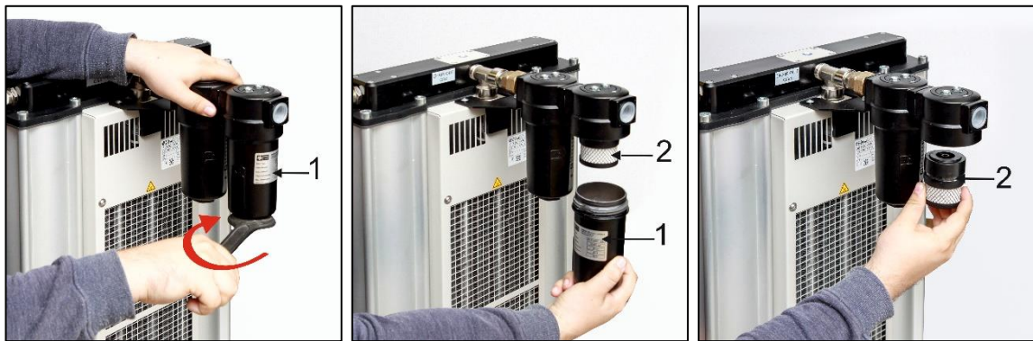
Fig. 24: Replacement of filter element in filter
